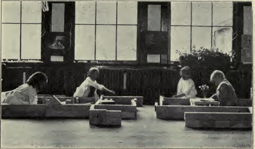
The Hill Floor Blocks at the Gregory Avenue School
